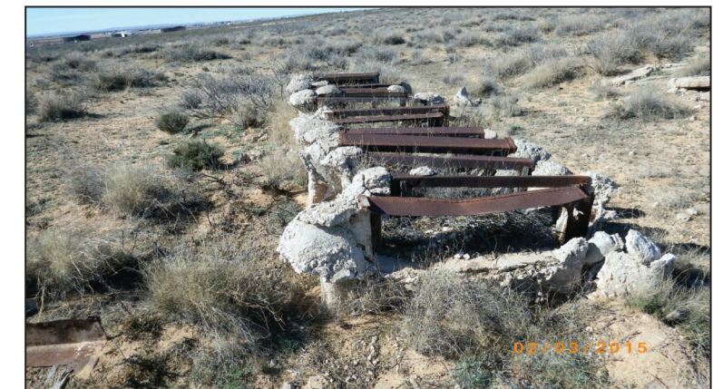
Figure 6. The row of individual sluice gates placed side by side looking northwest from the southeast end. Each metal frame represents a separate sluice gate.
