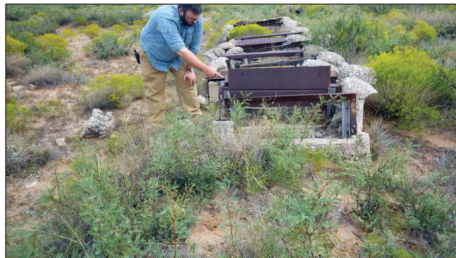
Figure 9. Nick Coleman pointing to a raised metal sluice gate at the northwest end of the row of sluice gate mechanisms.
