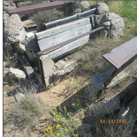
Figure 10. The two angle iron frames are shown in the center of the picture. A rectangular concrete block is inside the left end of the closer frame and two wooden sluice gate leafs are adjacent to the frames.
