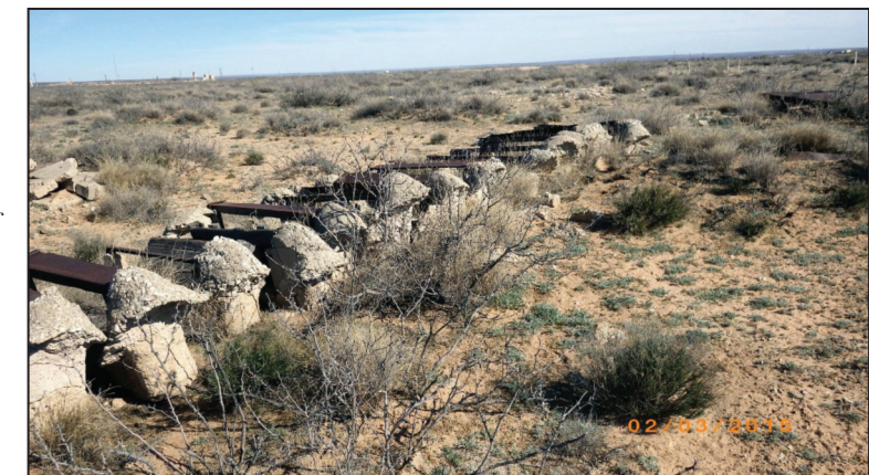
Figure 7. The concrete cylinders in the left foreground anchored one end of a sluice gate and a similar cylinder was on the opposite end of the metal frame. The cylinders were connected to a concrete tread on top of which the frame was mounted. View is to the southeast.
