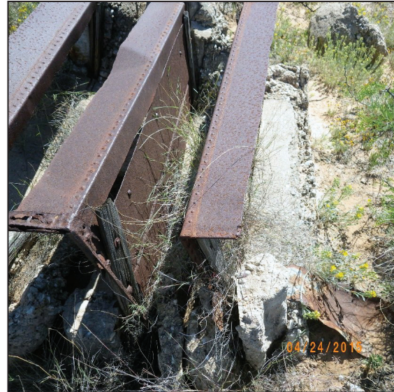
Figure 8. The metal knife gate in place with wooden slats at each end of the rectangular opening in the frame. The three bolts near the top of the gate must have held a piece of wood in place for use as a handle and probably to reinforce the gate.
