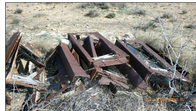
Figure 4. The central part of the southern 11 box frame pile. Wood is shown bolted to the short-sided face of several frames, but apparently the concrete part of the sluice gate had been removed or fell off.
